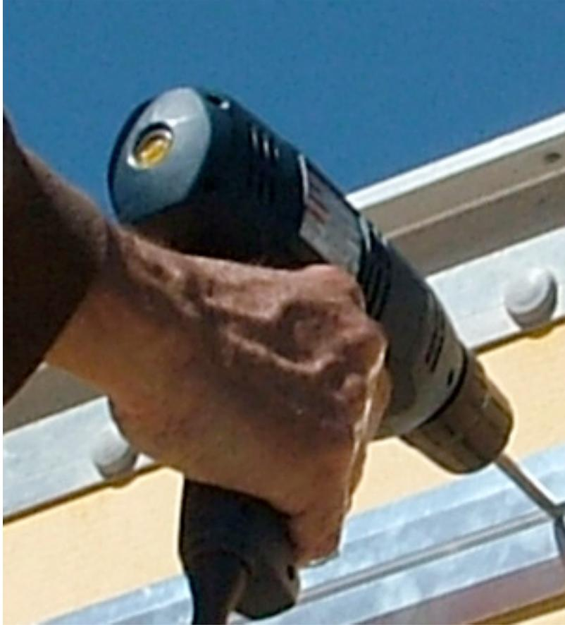
**Secure the base plate to the truck or wall with screws.**
